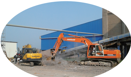
挖掘机开挖基槽
